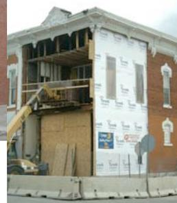
while the facade was partially deconstructed and then rebuilt from the ground up. Joel saved as much of the old facade as possible, matching new brick to the remaining historic materials, reusing the decorative stone window hoods, and repairing the metal cornice. New transom and storefront windows were installed. Inside, Joel saved the light fixtures and wood panels from the second floor office space and installed new sheetrock, flooring, and windows.
