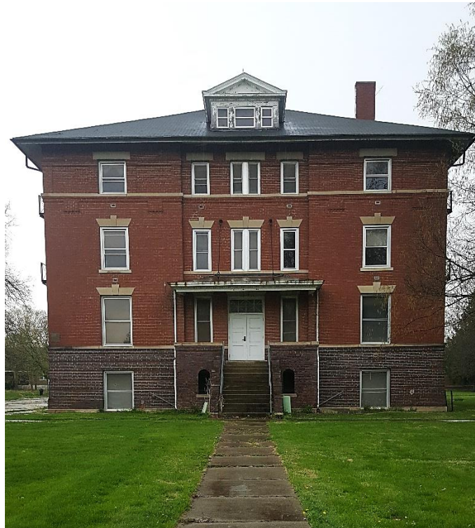
B-28 South Elevation & Main Entrance
