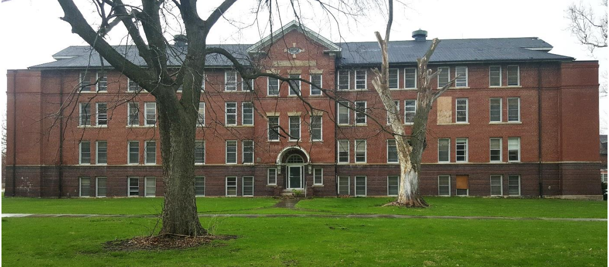
B-27 South Elevation & Main Entrance
