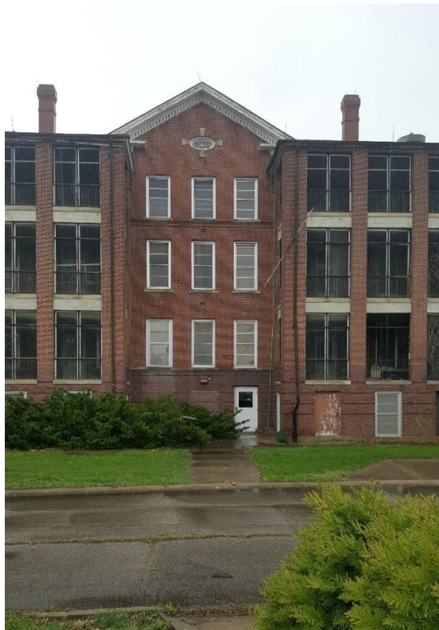
B-27 North Elevation (Partial View)
