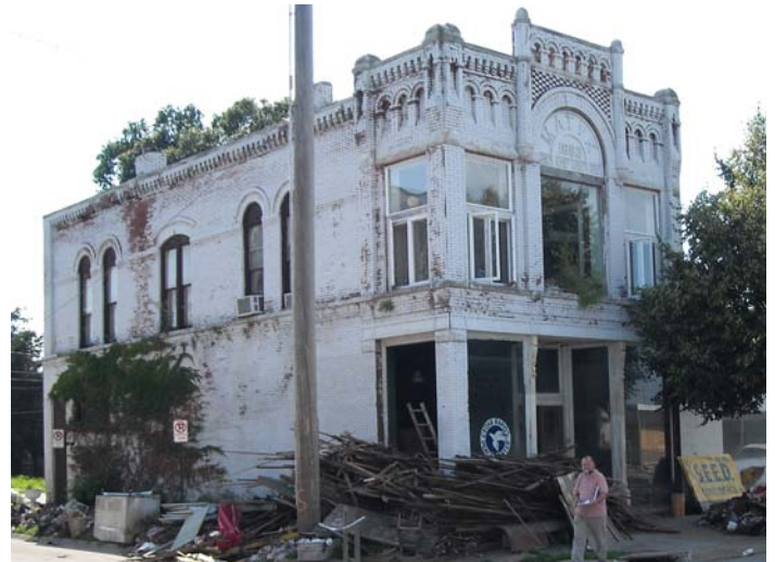
Historic Matyk Building in the Bohemian Commercial Historic District in Cedar Rapids.
