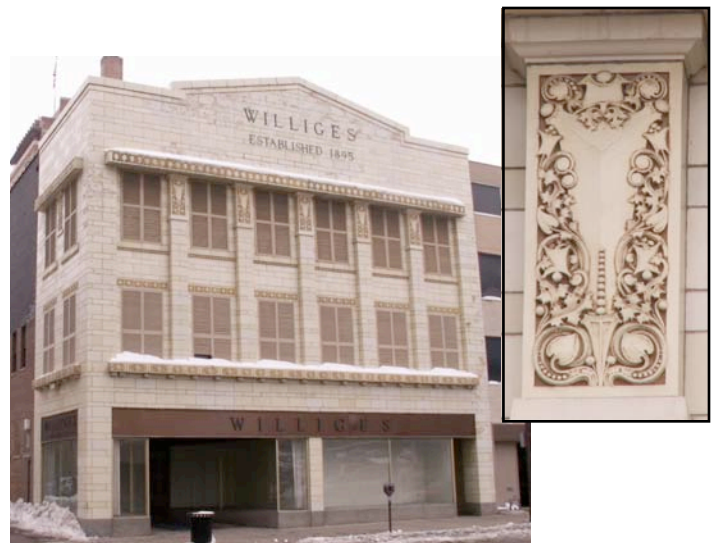
Williges Building, Sioux City, with detail of the terra cotta animal pelts. Photos courtesy the State Historical Society of Iowa's State Historic Preservation Office.
