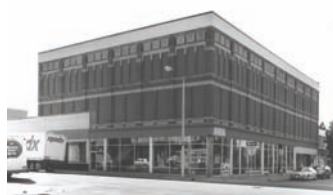
The Renaissance Revival
