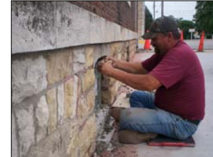
Masonry Repointing, Jewell
